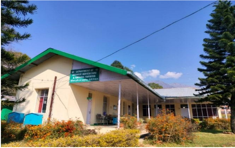
Renovated old Farm Building
